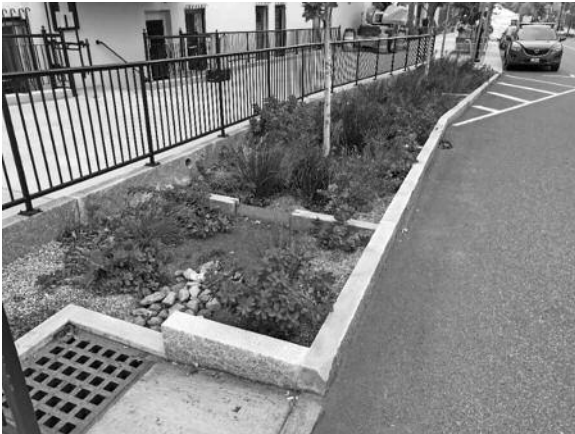
St. Paul bioretention system.
