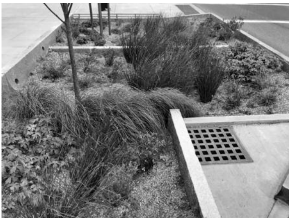
St. Paul Bioretention System Plantings Closeup
