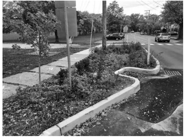
Locust St. Bioretention Nearing Completion
