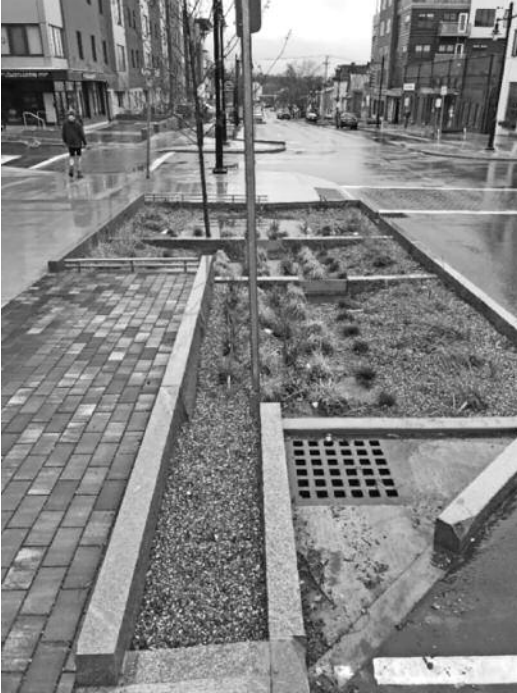
St. Paul newly installed pavers and newly planted bioretention system.
