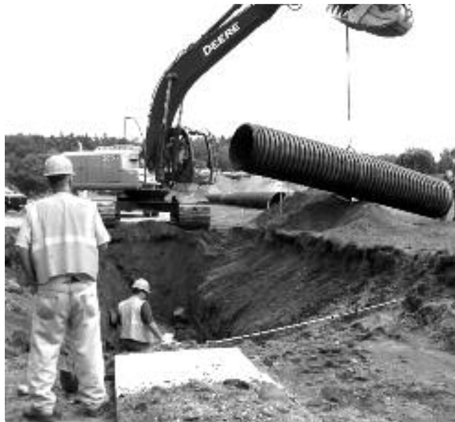
CP Smith storm drain installation
