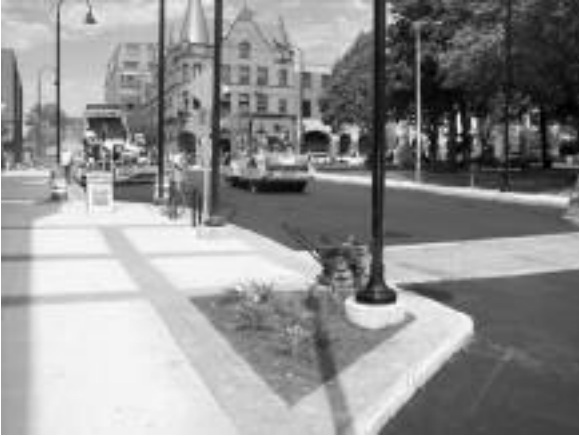
Putting finishing touches on St. Paul Street improvements
