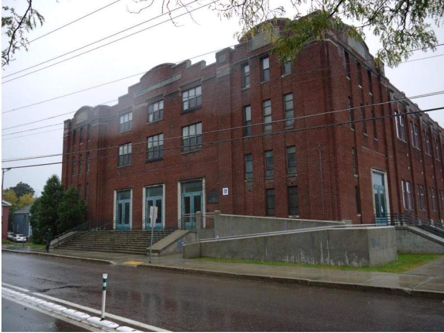
Accessible Ramp from South Union Street
