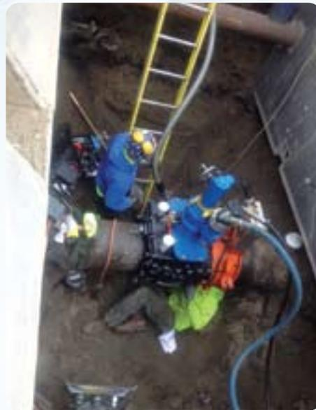
As part of our on-going investment into the infrastructure it is imperative that we can shut down water mains for servicing when breaks occur. This year we experimented with a valve that allows for installation under pressure. The picture above is of a 16 inch valve being installed on Lake Street. Another valve of similar design was installed on Main St at Battery.
