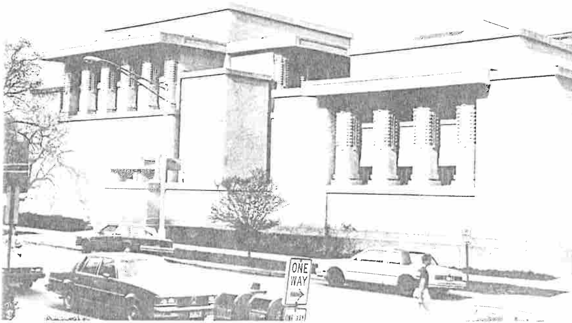
Fig. 14c. Once the repair work was complete, the entire building was sprayed with a concrete mixture consisting of pea-gravel, cement, and sand, which was then hand-
