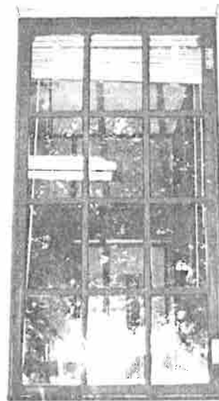
Fig. 6 f. View from the outside of the completely refurbished window. In addition to the steel repair and the installation of vinyl weatherstripping, the exterior was caulked with polyurethane and the single glass was replaced with individual lights of thermal glass. The repaired and upgraded windows have comparable energy efficiency ratings to new replacement units while retaining the historic steel sash, frames and subframes.
