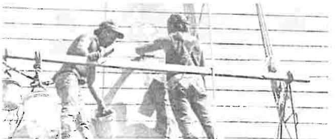
Fig. 13f. Workmen are applying patching concrete and using a trowel to form ridges to match the appearance of the historic concrete ridges that were originally created by the form boards.
