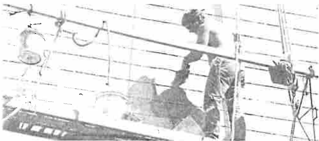
Fig. 13g. A soft brush is used to smooth the patch and to blend it with the adjacent historic concrete.
