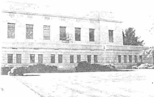
Fig. 6 a. View of the flanking wing of the State Capitol where the rolled steel casement windows are being removed for repair.
