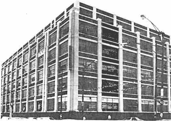
Fig. 10 a. A six-story concrete manufacturing building prior to the replacement of the steel pivot windows. Photo: Charles Parrott.
