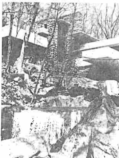
Fig. 5. "Fallingwater," near Mill Run, Pennsylvania (1936-37). This dramatic reinforced concrete residence by Frank Lloyd Wright is anchored into bedrock on the hillside and cantilevered over the stream. The great tensile strength of reinforced concrete made this type of construction possible. Photo: Paul Mayen.
