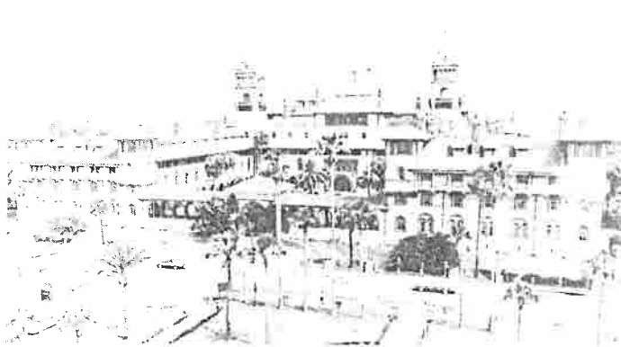
Fig. 3. Ponce de Leon Hotel, St. Augustine, Florida (1885-87). An example of unreinforced concrete used on a grand scale, this Spanish Colonial Revival hotel was designed by Carrere and Hastings and commissioned by railroad magnate Henry Flagler. The building now serves as the main campus hall for Flagler College. Photo: Flagler College.
