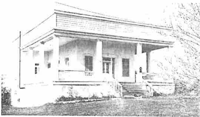
Fig. 2. Sebastopol House, Seguin, Texas (1856). This Greek Revival dwelling is one of the few remaining poured-in-place concrete structures in this Texas town noted for its construction of over 90 concrete buildings in the mid-nineteenth century. The high parapets surrounding the flat roof were lined and served as a water reservoir to cool the house. Photo: Texas Historical Commission.
