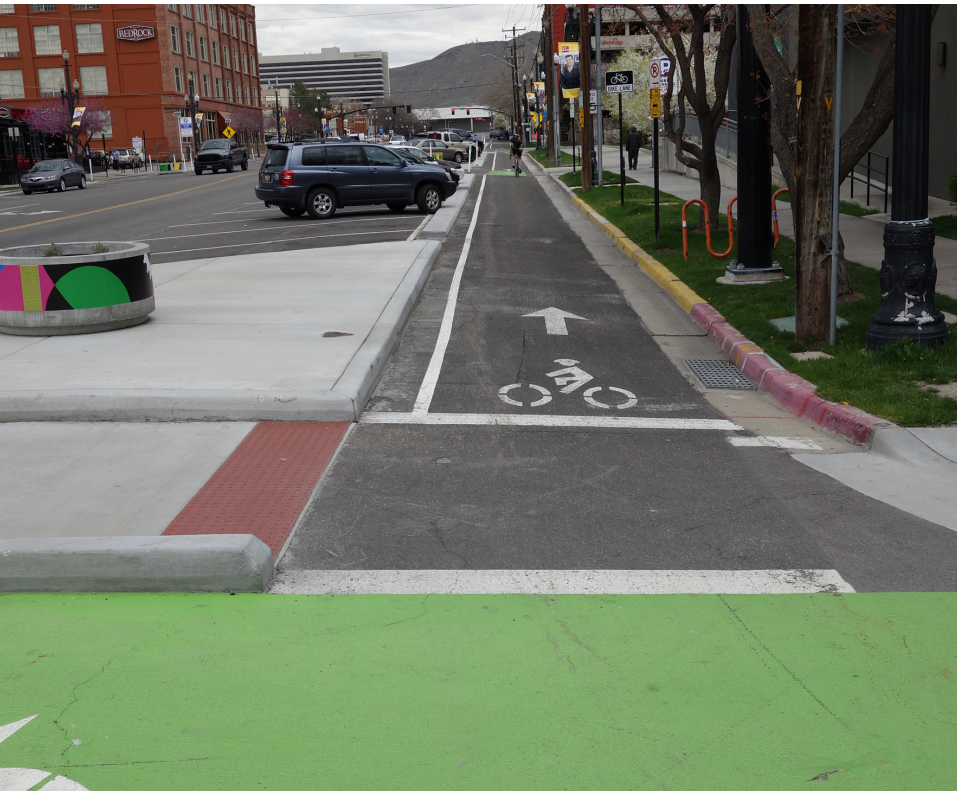
Protected intersection for bike lanes in Salt Lake City. Item B in the concept on the next page.
