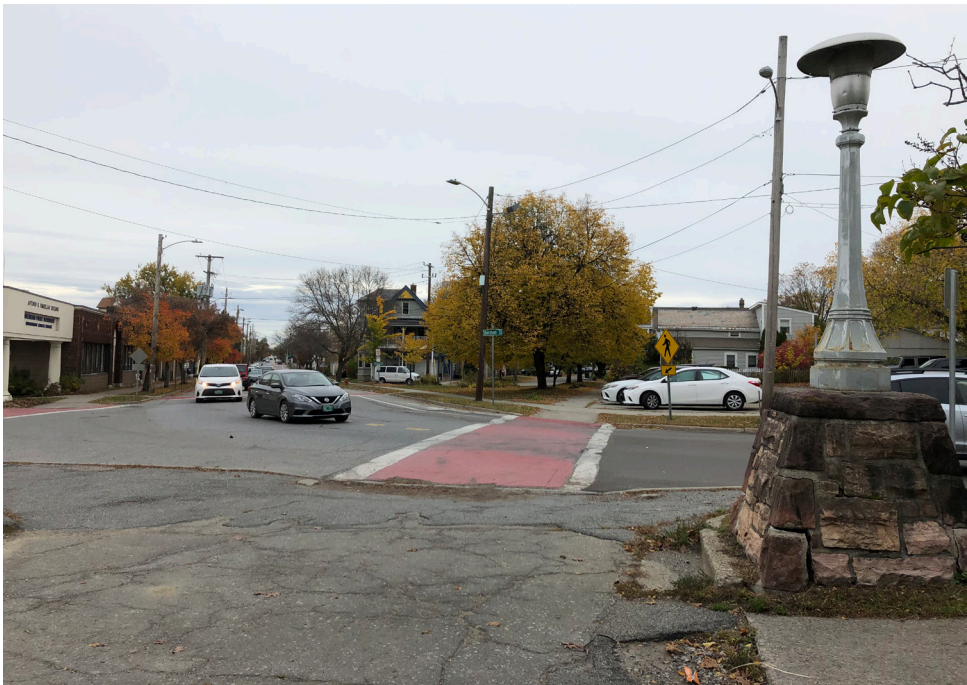
The North Avenue intersection with Sherman Street and Battery Park is wide and lacks high visibility crossings, detectable edges at each curb ramp, and smooth pavement at the entry to Battery Park.
