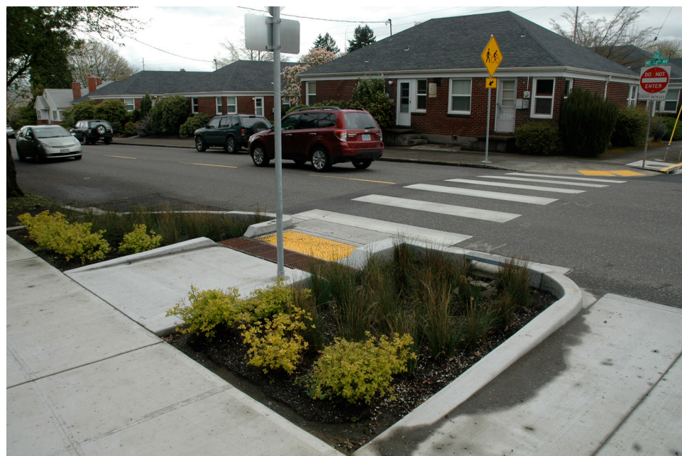
Stormwater Curb Extension in Portland, OR
