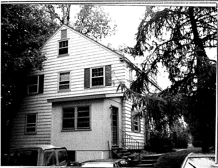
Rear View 201 So. Prospect St. Burlington, VT
