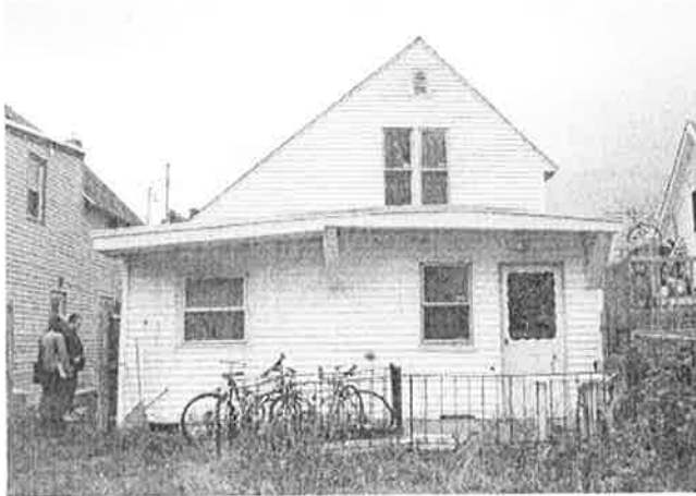
Rear elevation, showing non-historic rear addition.
