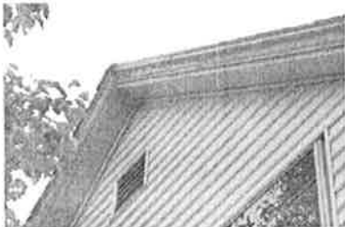
The molded cornice is one of few remaining historic elements.
