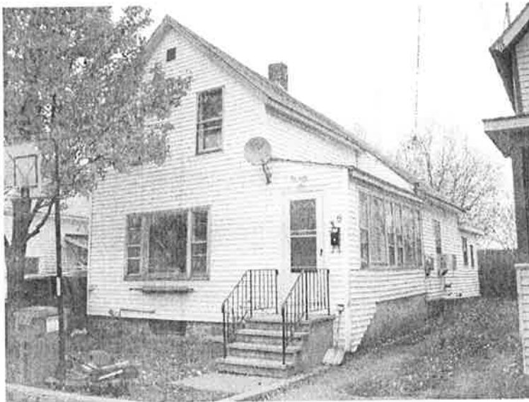
View of front elevation looking easterly.
