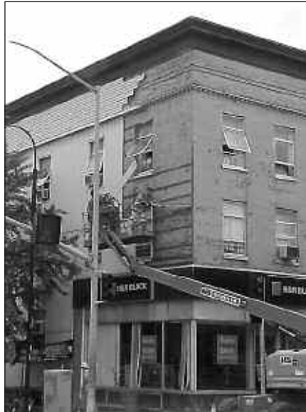
Work performed at 207-217 College Street.
