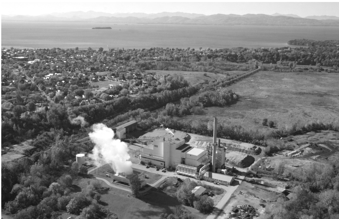
Aerial view of McNeil plant
