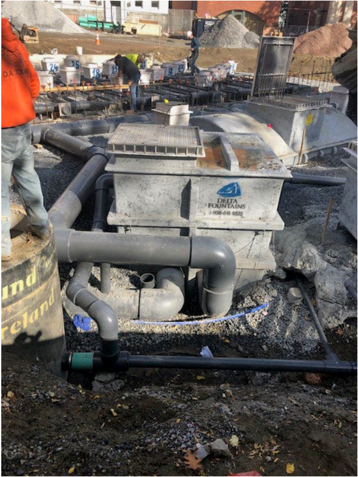
Connection to SMH #1
