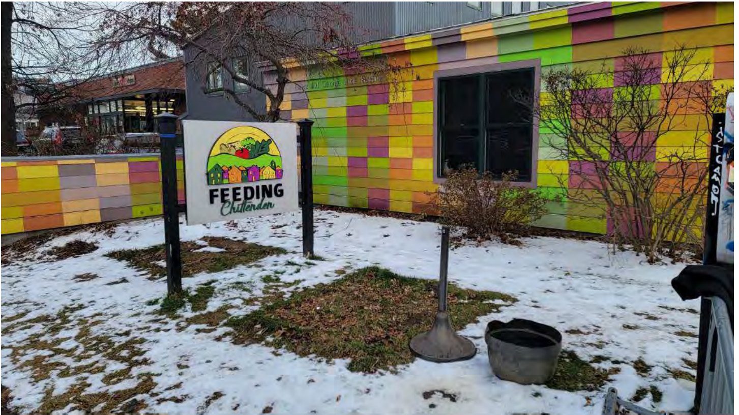
Front of the building - Location of addition.
