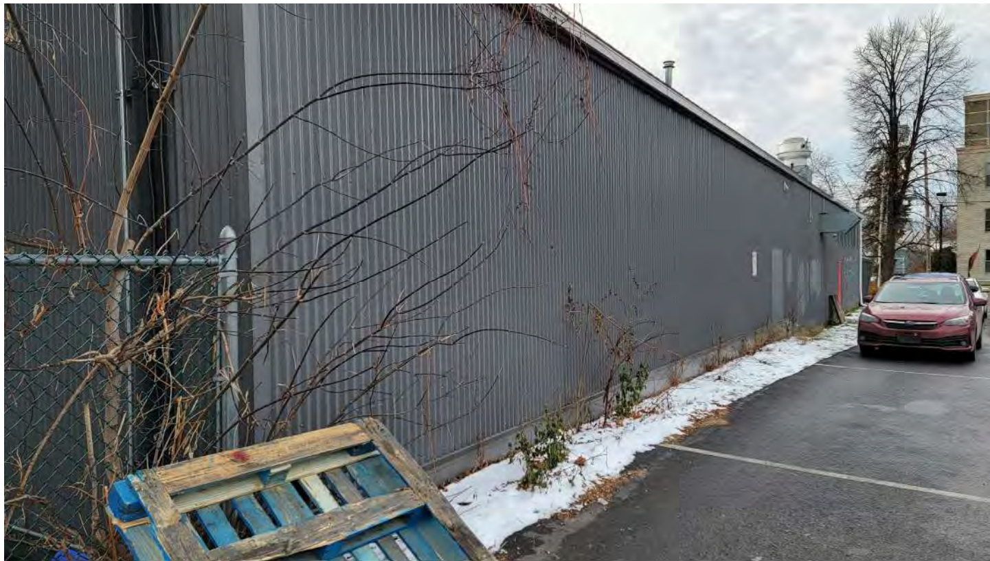
North side of the building.
