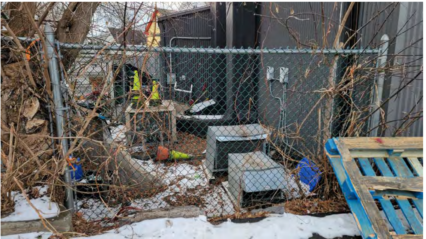
Rear of the building.
